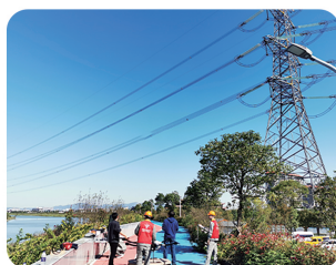
Power Grid Inspection
